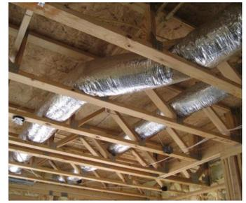
*Ducts are run straight and supported properly.*
