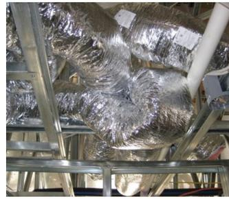
*Ducts are crammed into cavity, kinked and sharply bent.*
